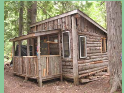
Consultation with this cabin user’s group, whose cabin is on Atco’s operating area, resulted in a strategy to retain timber around the cabin, as well as the re-location of a planned haul road.
