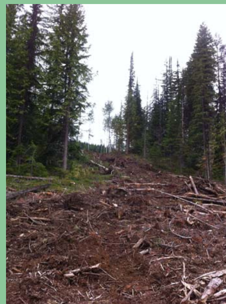
Deactivation of skid trails including this one shown was found to effectively manage erosion potential and also re-store soil productivity. Following deactivation, trails are re-planted.
