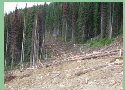
Atco rehabilitates unneeded roads by complete recontouring. This is done to minimize the losses of productive forest land to roads and to reduce the risk of future landslides and soil erosion resulting from bare road surfaces.
